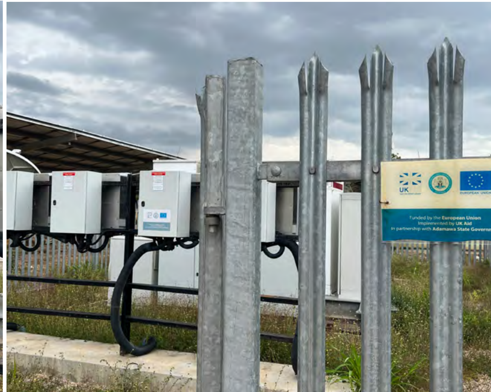
TESLA Power Packs and Remote Monitoring System installed at the General Hospital, Mubi, Adamawa State under the 11th EDF-Nigeria Energy Support Project (NESP)/Solar Nigeria
