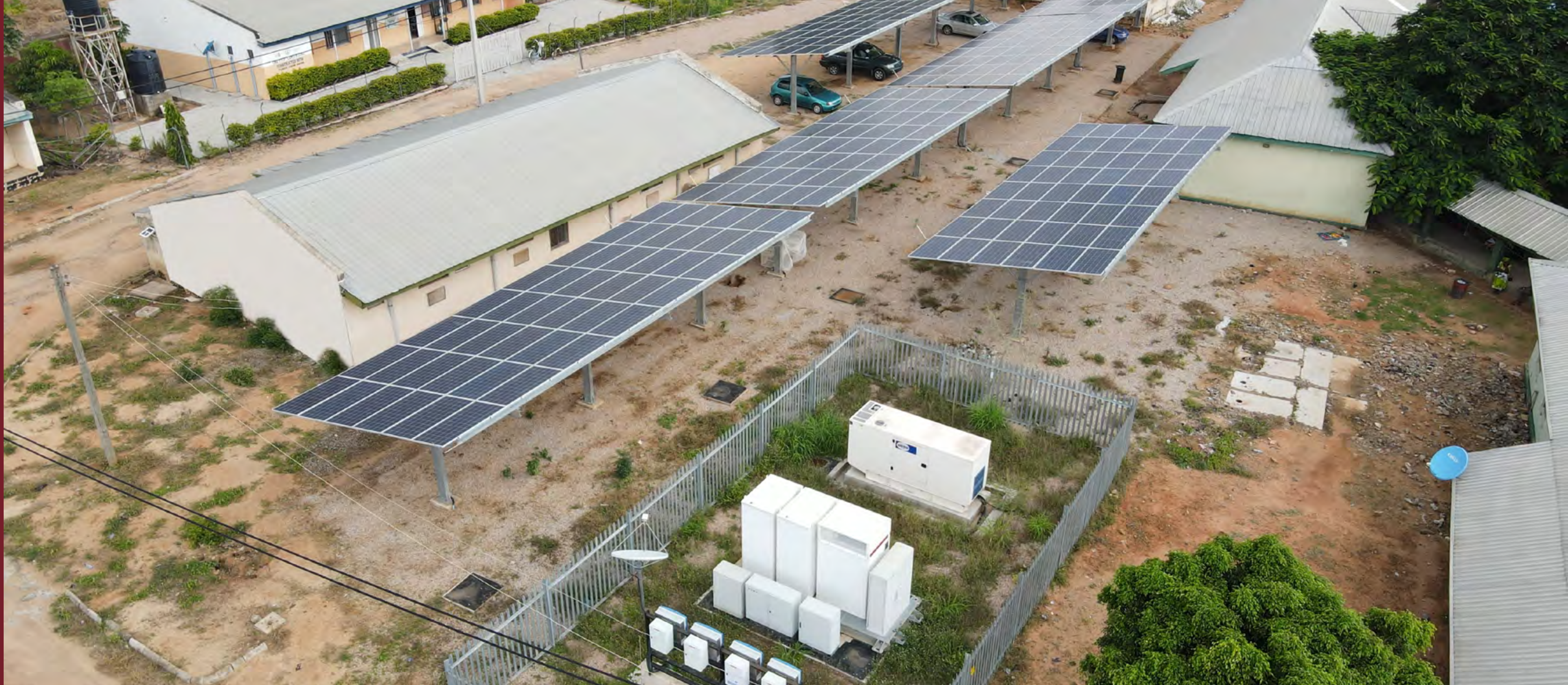
104 KW Off-grid Solar Photovoltaic (PV) System installed at the General Hospital, Mubi, Adamawa State under the 11 th EDF-Nigeria Energy Support Project (NESP)/ Solar Nigeria
